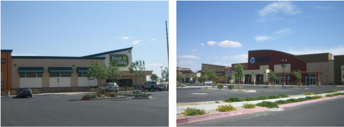
Figure 9.04-E: An example of dynamic roof lines
