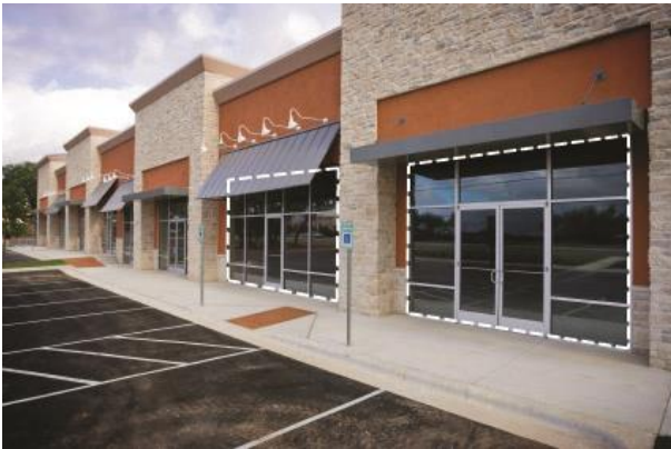
Figure 12.07-J: The window area is illustrated within the dashed line area for the two storefronts in the above image.
