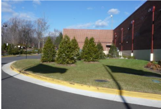
Figure 10.08-A: The above image illustrates a vegetative screen that hides HVAC equipment and a dumpster.
