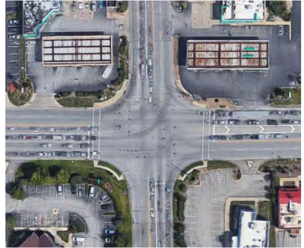
ABOVE: South Avenue and US-224. Google Maps, 2019.
