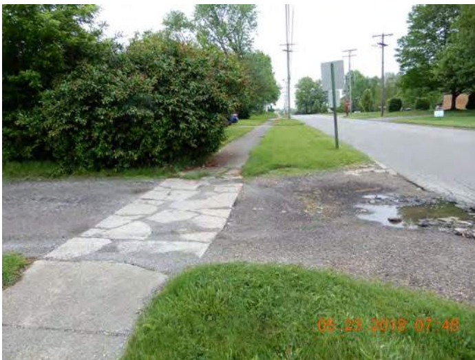
A section of badly broken sidewalk near Stadium Drive Elementary. D'Avignon, 2018.
