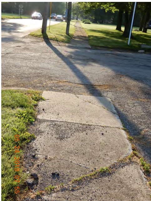
The sidewalk is in poor condition and does not have marked crosswalks or ADA compliant curb ramps.
