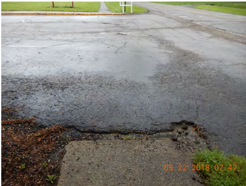
The above sidewalk has been cut in half by a driveway. It is not ADA accessible or visible to entering busses or vehicles. Signage is not present to show the crossing.
