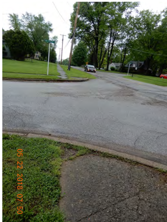
The sidewalk does not feature ADA compliant curb ramps or tactile pavers. The crosswalk itself needs to be painted and signage should be installed to alert drivers to its location.
