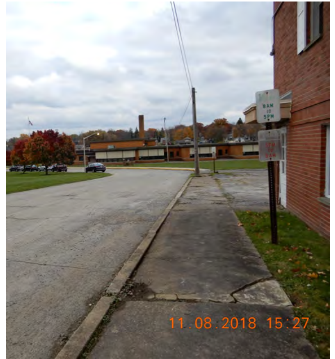
Sidewalks in the area directly surrounding the school are in poor condition and desperate need of repair.
