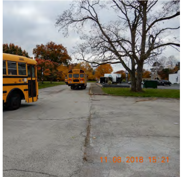
Lack of ADA curb ramps, marked pedestrian crossing with signage, or pavement markings
