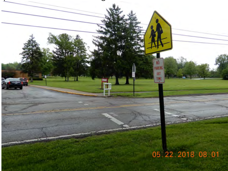
This crosswalk is faded, does not have ADA-compliant curb ramps, and the nearest end of the crosswalk empties out onto the grass.
