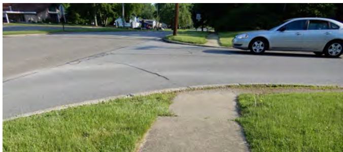
Crosswalks are faded on Glenwood Ave. and missing ADA compliant curb ramps
