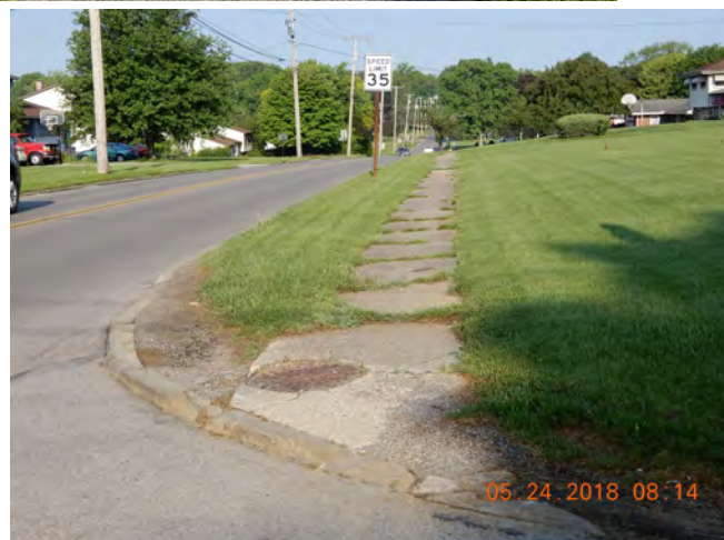
Crosswalks should be repainted with high visibility markings and new ADA compliant curb ramps installed at intersections near the school.
